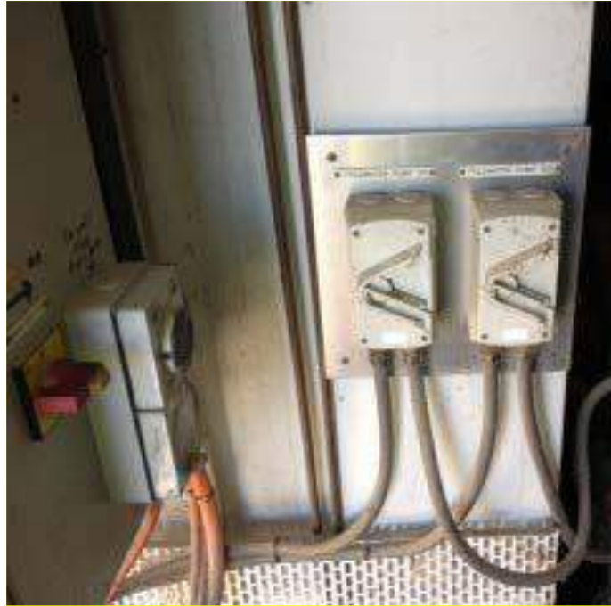
Figure 10 - Control Switches on Side of Boiler
