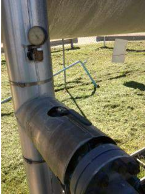
Figure 7 - LPG Tank Control Valve Located on the Bottom Side of the Tank
