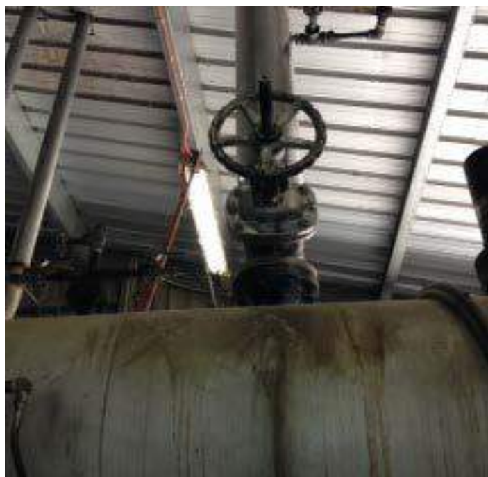
Figure 11 - Control Valve on Top of Boiler
