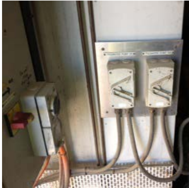
FIGURE 10: CONTROL SWITCHES ON SIDE OF BOILER
