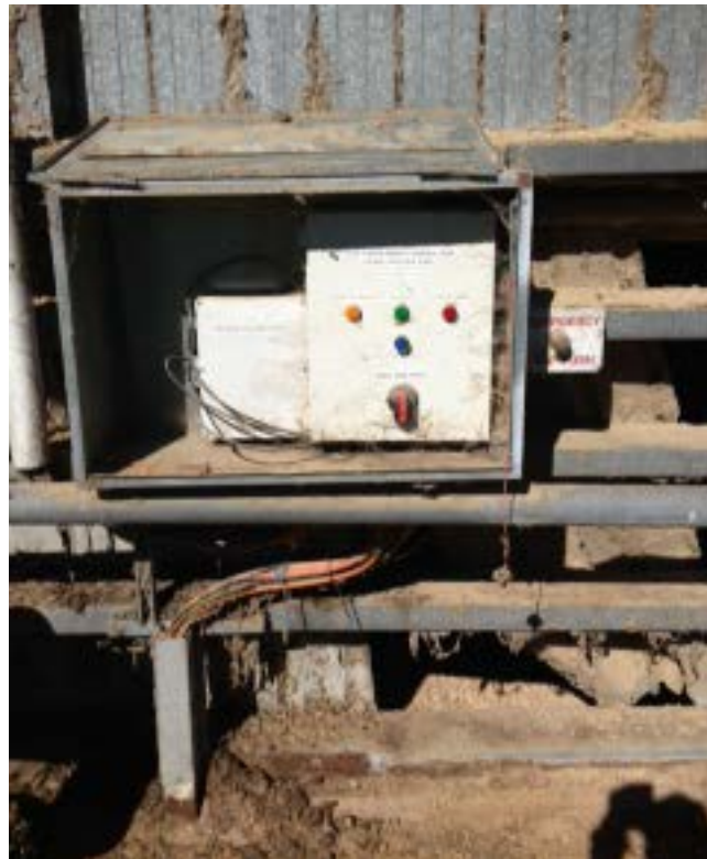
FIGURE 8: CONTROL PANEL IN COMMODITY SHED
