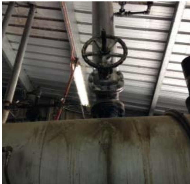
FIGURE 11: CONTROL VALVE ON TOP OF BOILER
